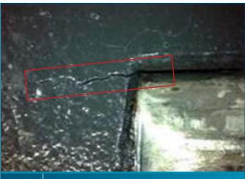
Crack width is less than or equal to 0.2 mm.
